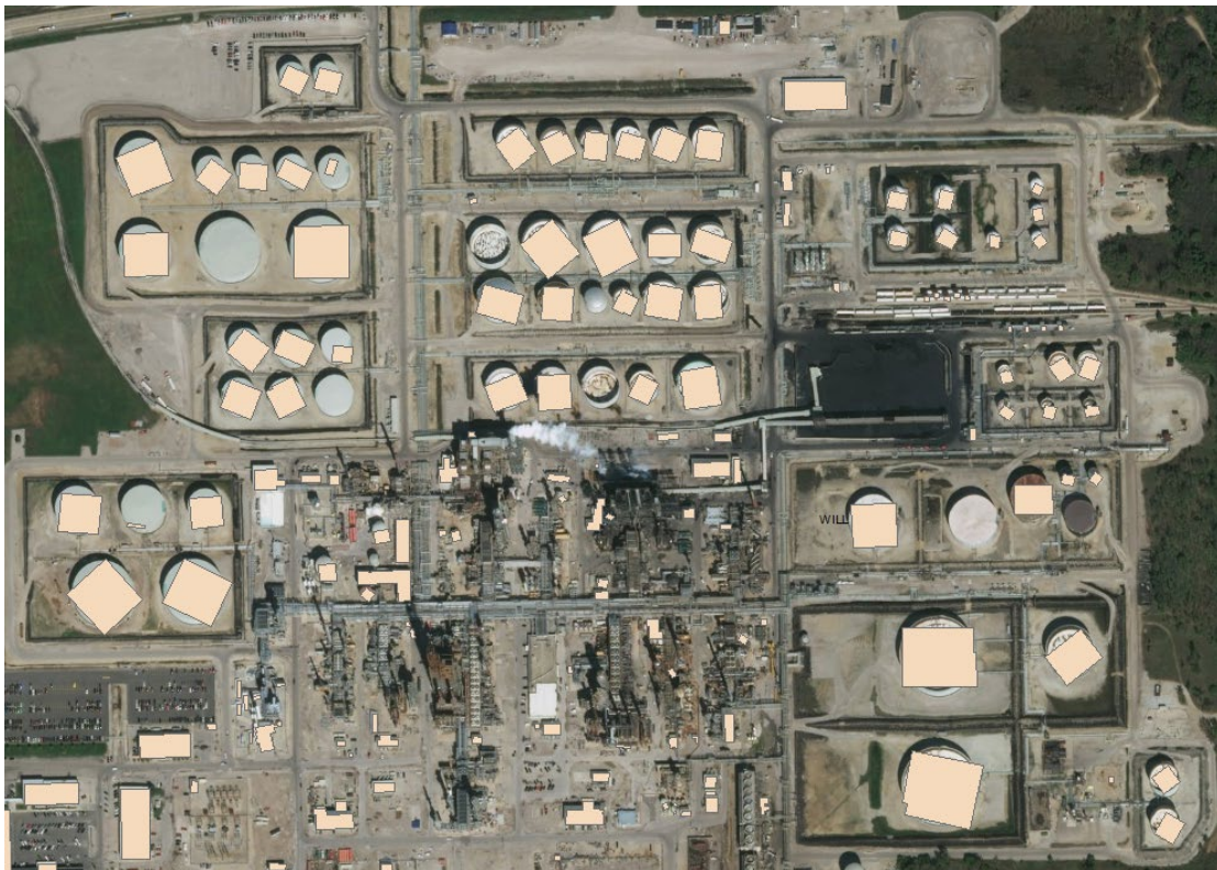
Figure 2. A sample dataset showing errors from squaring buildings from Will County, Illinois
