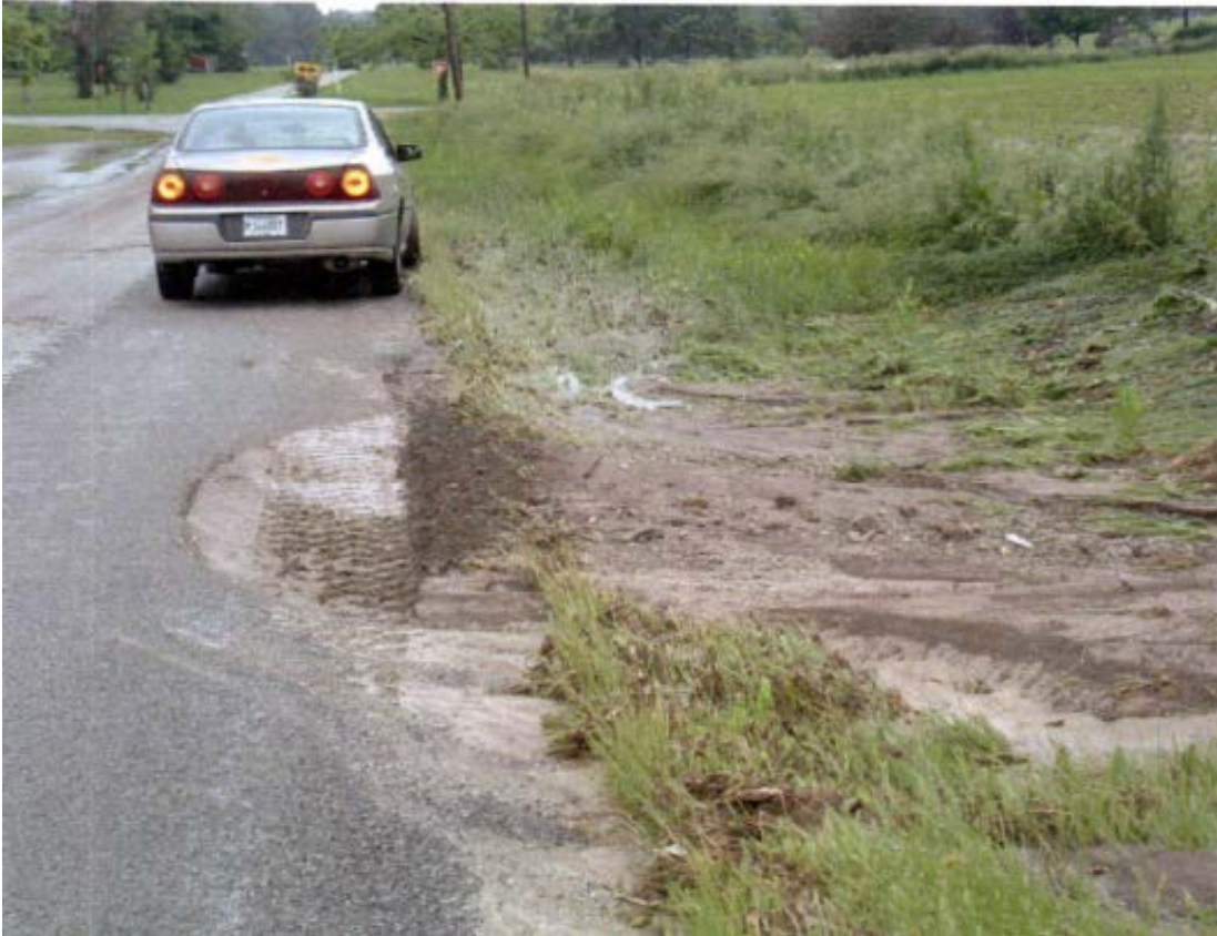
Sediment on the road shows runoff during flood events from adjacent farm fields
