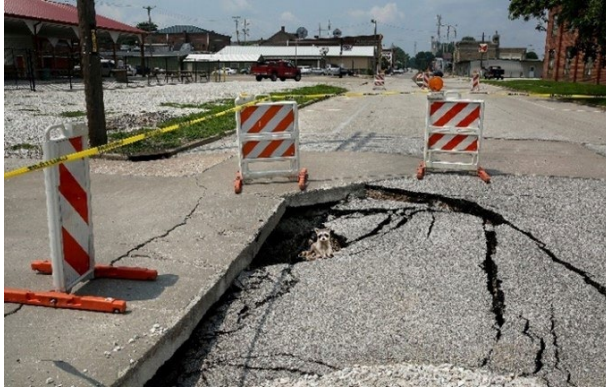
Figure 29. A sinkhole caused by the April 2013 floods at the intersection of E Main St and Monroe St in Beardstown, which connects the two grain elevators in town. Farmers were delayed by this road closure. Credit: Peoria Journal Star
