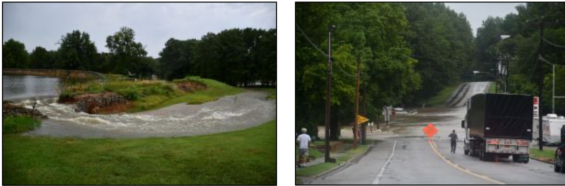
Figure 30. A six-foot breach on the Nashville Reservoir's secondary dam (L) and resulting flooding on IL Route 15 (R). Source: Charles Guffey, The Nashville News .
